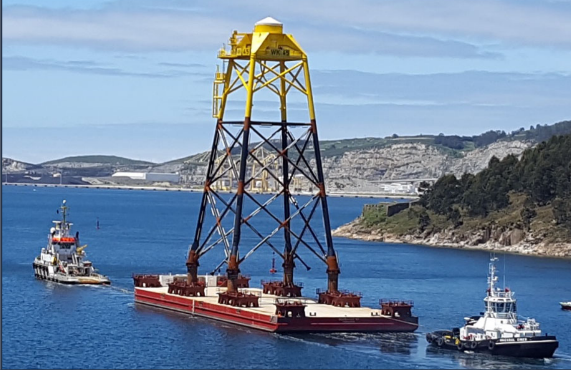
Figure 3.3-2 Foundation Transportation and Installation
