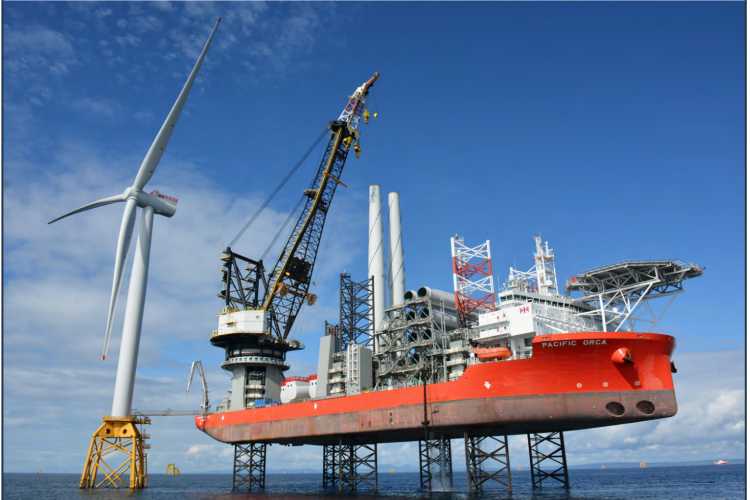
Figure 3.2-2 Wind Turbine Generator Installation
