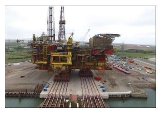
Figure 17. Skidding Brent Delta topside onto Able Seaton Port (Shell 2019)
