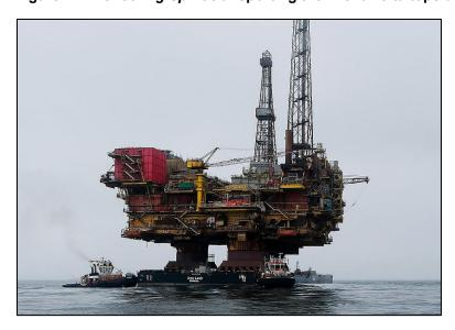
Figure 15. Iron Lady barge transporting the Brent Delta topside (Shell 2017b)
