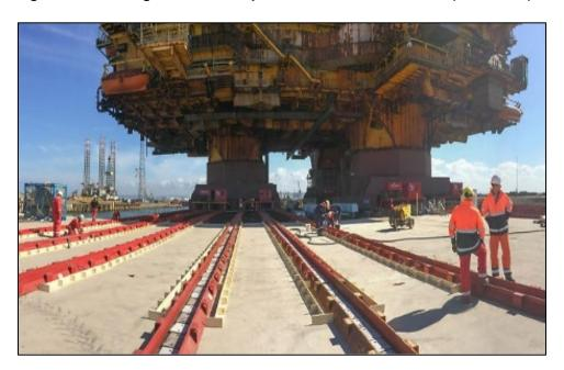
Figure 18. Skidding Brent Delta topside onto Able Seaton Port (Shell 2019)
