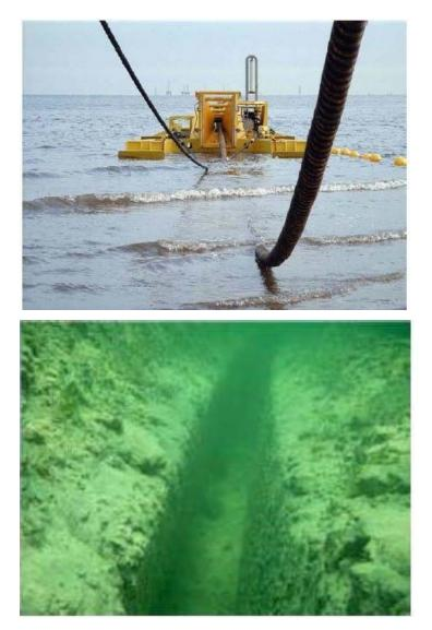
Figure 4-2. Cable-pulling vessels.
