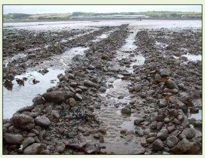
Figure 5.4: Physical impacts of export cable installation on the lower shore at Robin Rigg Offshore Wind Farm
