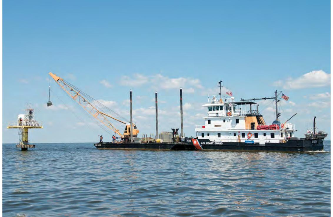
Crewmembers aboard Coast Guard cutter Sledge use the ship's crane to lower a new transformer down to Craighill Entrance front range light Aug. 25, 2014. Crew members from Aids to Navigation Team Baltimore help guide the transformer onto the structure by use of the tag line.
