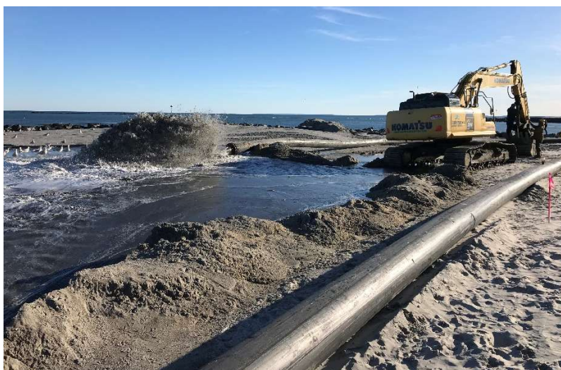
Figure 4-3. Beach nourishment at Hampton Beach State Park using dredged material from Hampton-Seabrook Harbor (November 23, 2019). The sand was pumped onto the beach via a pipeline (left photograph). Photograph on the right is a close-up of sand discharged from the pipe.
