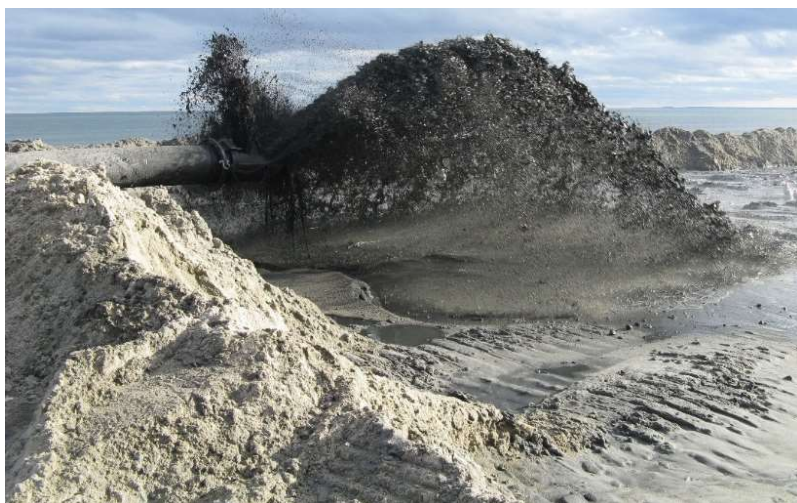
Figure 4-2. Beach nourishment at Seabrook Beach using dredged material from Hampton-Seabrook Harbor (December 11, 2012). The sand was pumped onto the beach via a pipeline (left photograph) and then graded with a bulldozer (right photograph).
