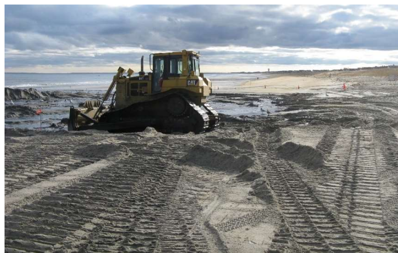
Figure 4-2. Beach nourishment at Seabrook Beach using dredged material from Hampton-Seabrook Harbor (December 11, 2012). The sand was pumped onto the beach via a pipeline (left photograph) and then graded with a bulldozer (right photograph).
