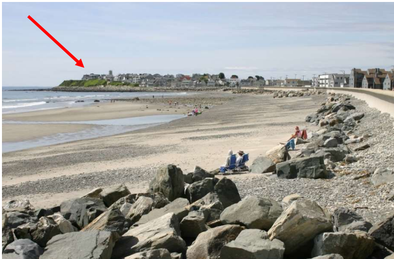
Figure NB-3. North Beach looking south on June 6, 2019. Great Boars Head (arrow) forms its southern boundary. A cement seawall extends the entire length of the beach. Note the riprap at the base of the seawall placed to diminish wave impact and the megacast platform.
