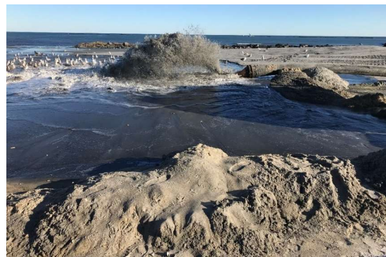
Figure 4-3. Beach nourishment at Hampton Beach State Park using dredged material from Hampton-Seabrook Harbor (November 23, 2019). The sand was pumped onto the beach via a pipeline (left photograph). Photograph on the right is a close-up of sand discharged from the pipe.
