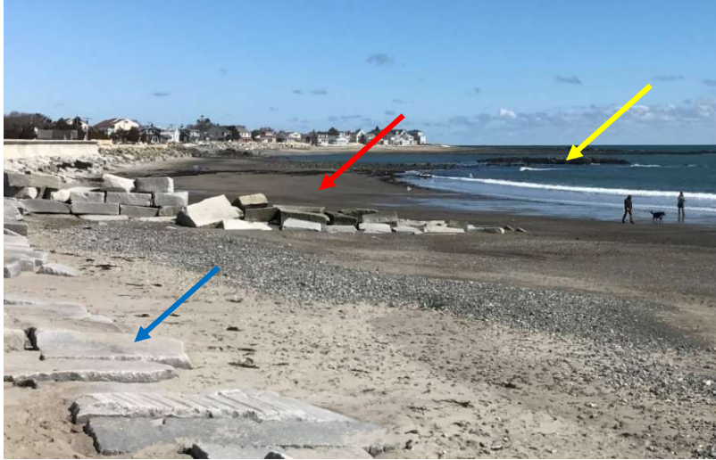
Figure NB-2. Photograph of the northern headland at North Beach taken on March 18, 2017 from station NB01. Note the stone groin in the foreground (red arrow), stone blocks at the base of the seawall (blue arrow), and a megacast platform at the northern end of the beach (yellow arrow).
