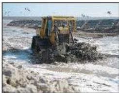
Bulldozers move sand as it gets pumped onto the beach at the Caminada shoreline projects at Port Fourchon.
