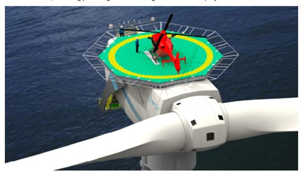
Another unique and leading development was under the 2B Energy, where Jakobsson led development with the HCA (Helicopter Certification Agency) and the CAA (Civil Aviation Authority) to develop process and design for secure and approved landing of helicopter on wind turbines and the design of helideck (see illustration above). This was undertaken in close collaboration with expert pilots from the leading UK offshore helicopter operations companies.
