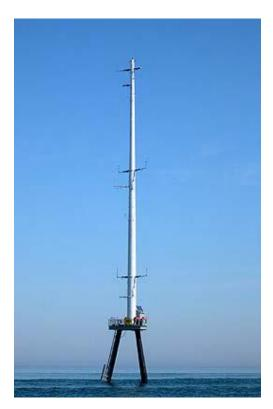
Figure 3-5. Example of Monopole-mast Meteorological Tower
