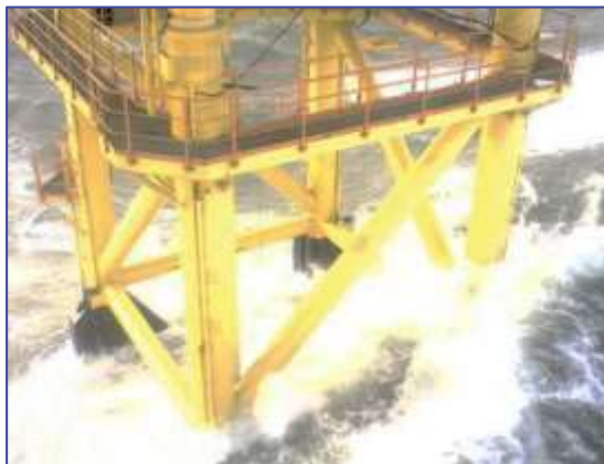
Breaking wave at FINO-1 platform in 28m water depth when significant wave height is only 6 m
