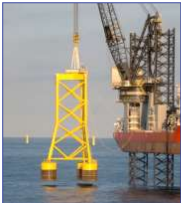
First prototype suction-bucket jacket at Borkum Riffgrund I, pioneered by Orsted
