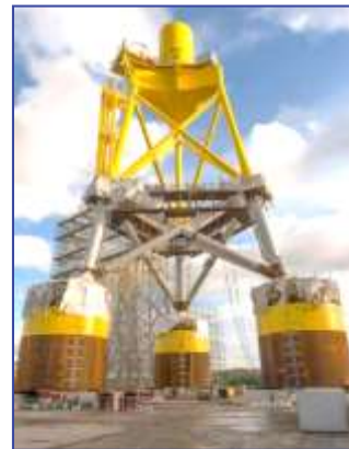
Suction-bucket jacket ready for European Offshore Wind Deployment Center
