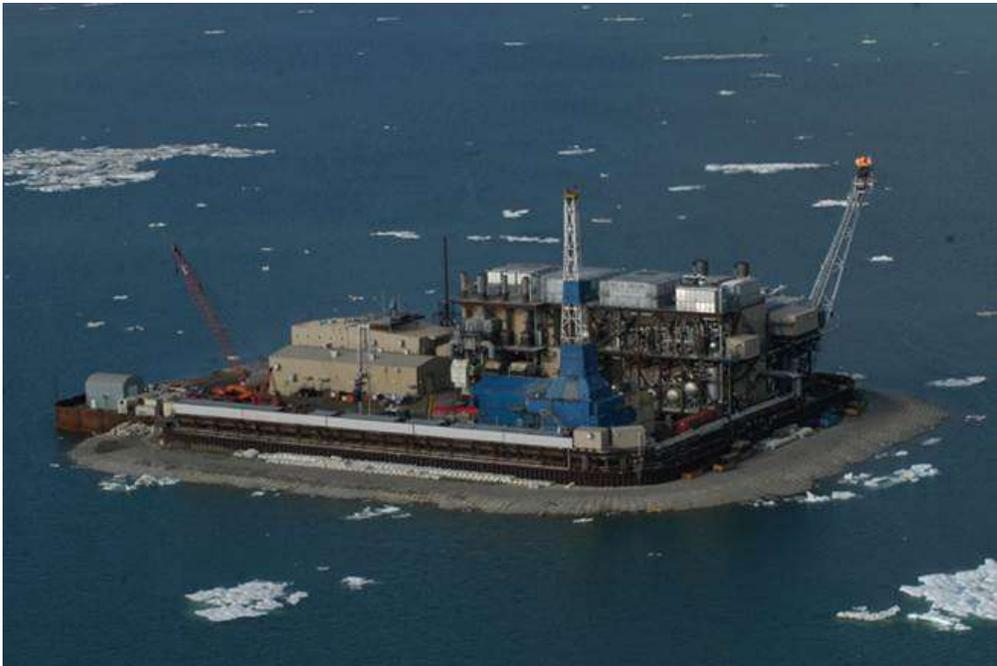
Figure 1.6. Northstar production site in Alaska operated by Hilcorp Alaska, LLC. Northstar is located on an artificial island. It is located 6 miles offshore in water that experiences significant ice formation. Product flows through a subsea pipeline. Source: <http://libertyprojectak.com/>
