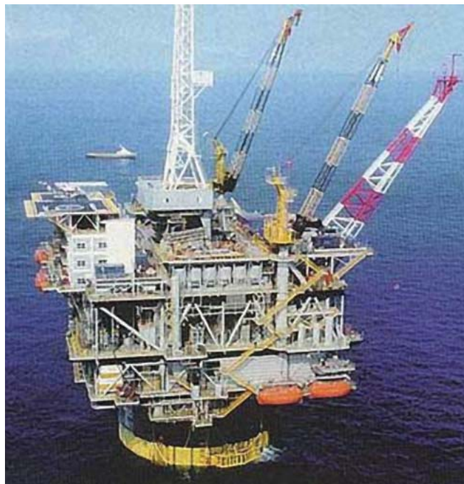
The spar structure Genesis, owned by Chevron/Texaco, operates in a water depth of 2,590 feet in the Gulf of Mexico.
