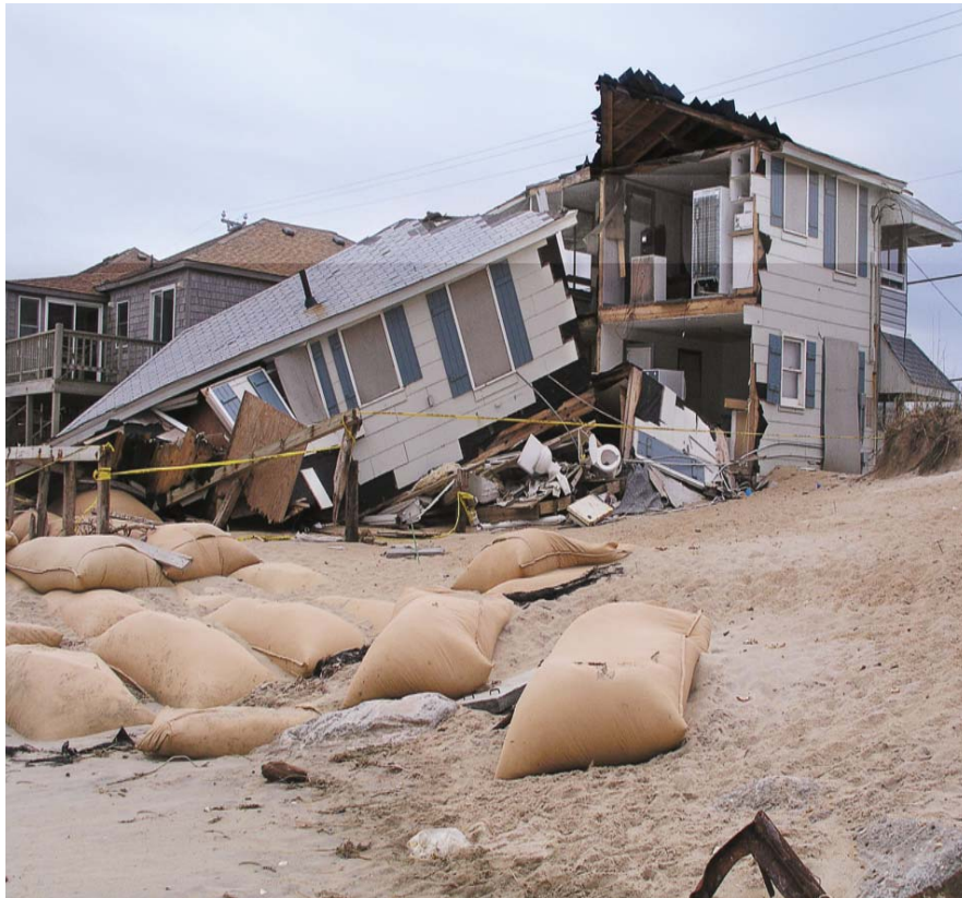
The power of Hurricane Katrina was evidenced throughout the Gulf Coast Region.
