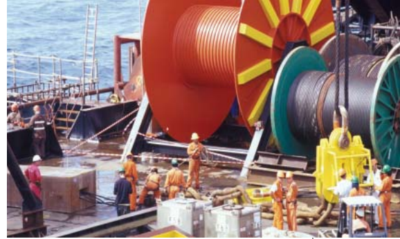
Below bottom: A stack of pipeline that will be used to transport gas and oil from the development field to shore. The pipeline diameters are 16, 20, 24, and 28 inches.
