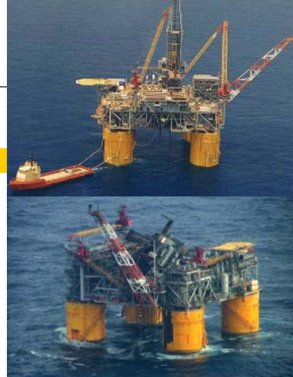
The Shell Mars platform before and after Hurricane Katrina in September 2005.
