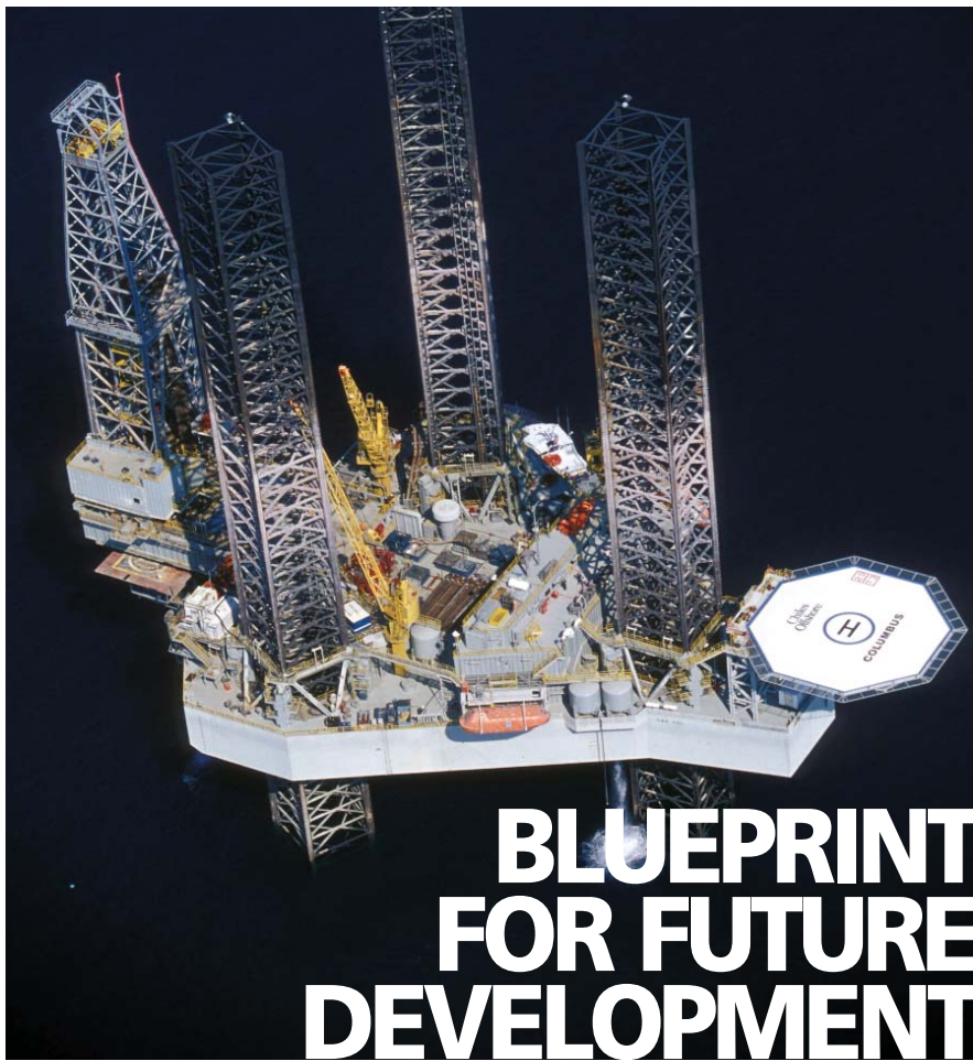
Left: A jack-up rig used to drill for oil and gas on the Outer Continental Shelf.
