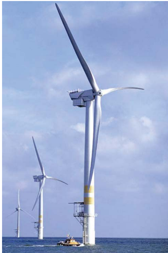
Inspecting an offshore windfarm, Arklow Bank, Ireland. Photo courtesy of GE Energy.
