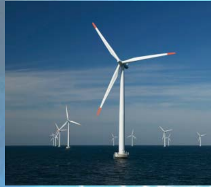
Wind turbines in Nysted Offshore Windfarm, Denmark. Photo courtesy of Nysted Havmøllepark.
