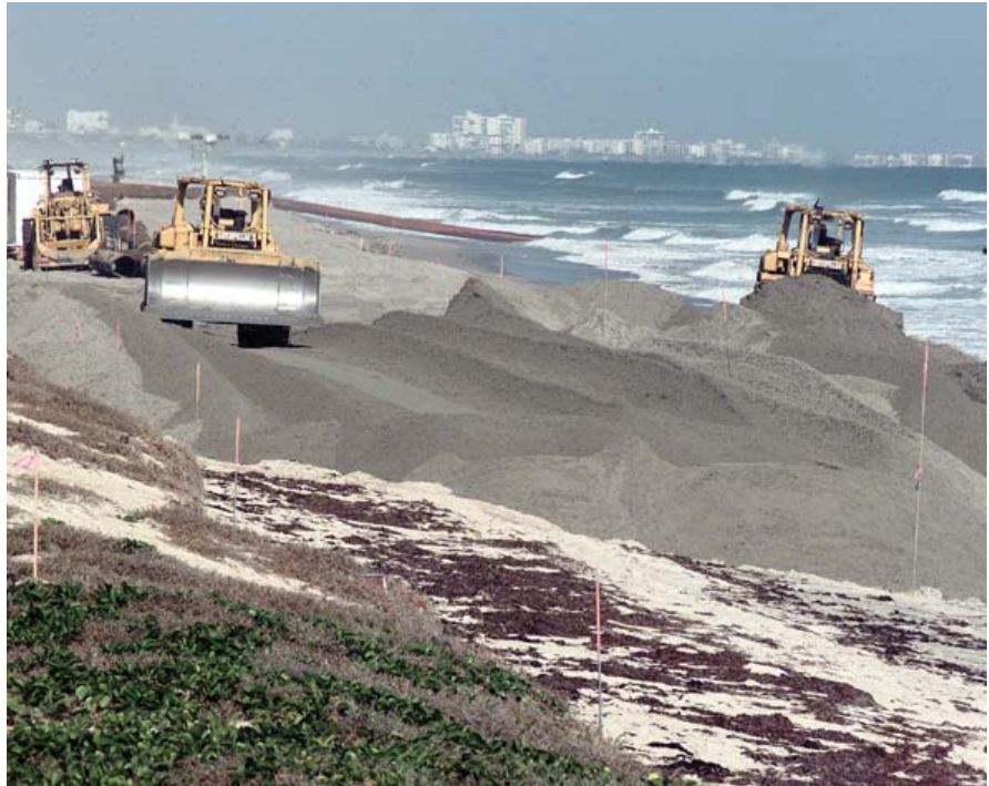
Above: The MMS also signed a Memorandum of Agreement with the U.S. Air Force to provide up to 350,000 cubic yards of Federal sand to restore the Atlantic shoreline of Patrick Air Force Base, in Brevard County. The sand was dredged from Canaveral Shoals, then transported to the project sites and hydraulically pumped from the dredge ship. This project was completed on April 29, 2005.
