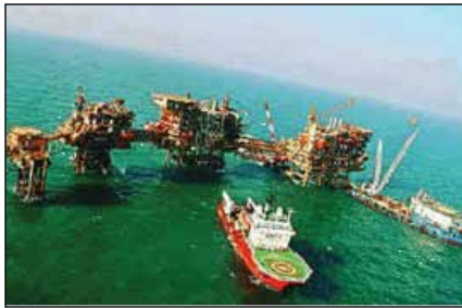
The Mumbai High North platform.
